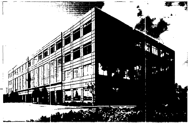
Lakeside II, Flagler Center Jacksonville, FL
