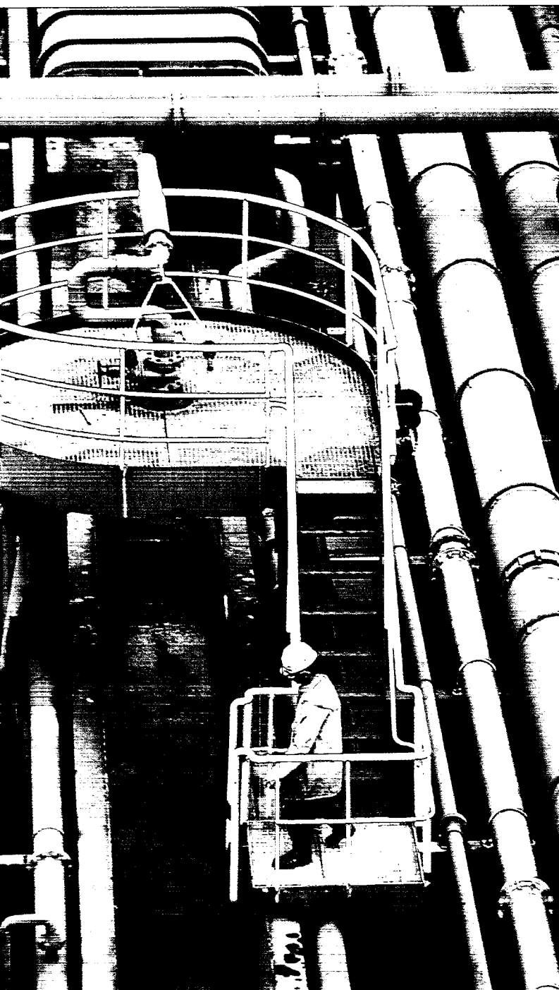
In Vietnam, ConocoPhillips is a major acreage holder with more than 3 million net acres under license. The company installed two new wellhead platforms at the Rang Dong field (above) in 2002, increasing field production by 80 percent.
